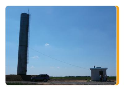
In Miratorg's case, each building has its own autonomous water supply system, including a water tower and an area where the automation control system is located, along with the water distribution system.
